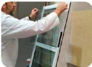
APPLY THE WINDOW FILM
