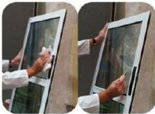
CLEAN THE SURFACE
