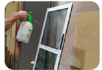
SPRAY THE SURFACE WITH WATER
